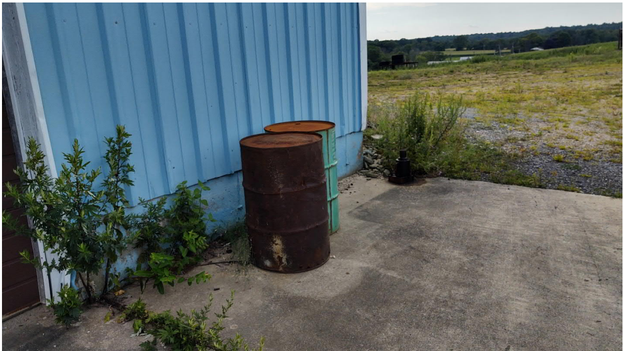
Photograph 4 Unknown Drums in Poor Condition
