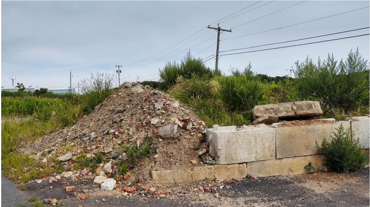
Photograph 11 Soil and Demolition Debris at Landscaper Building
