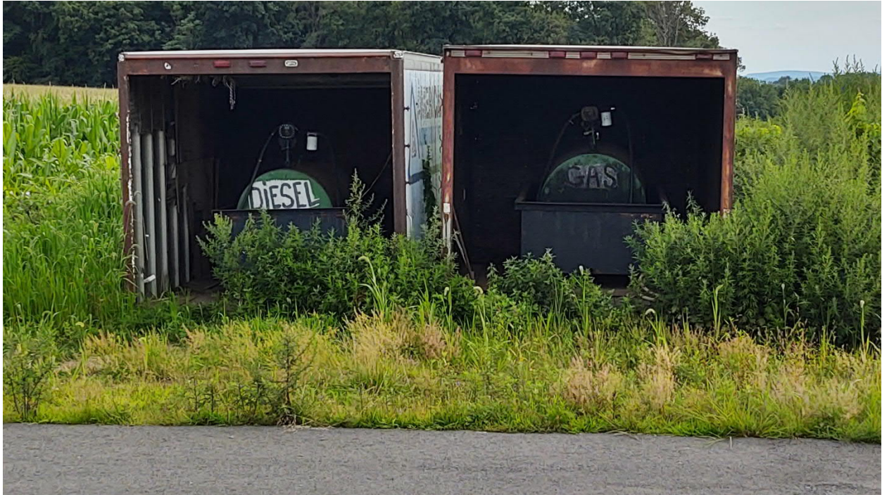
Photograph 1 Diesel and Gasoline Storage Tanks
